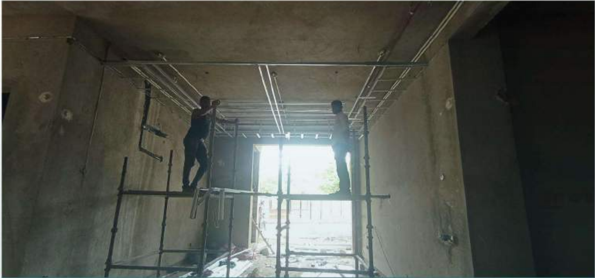
POP FALSE CEILING WORK AT SAMPLE FLAT TOWER B
