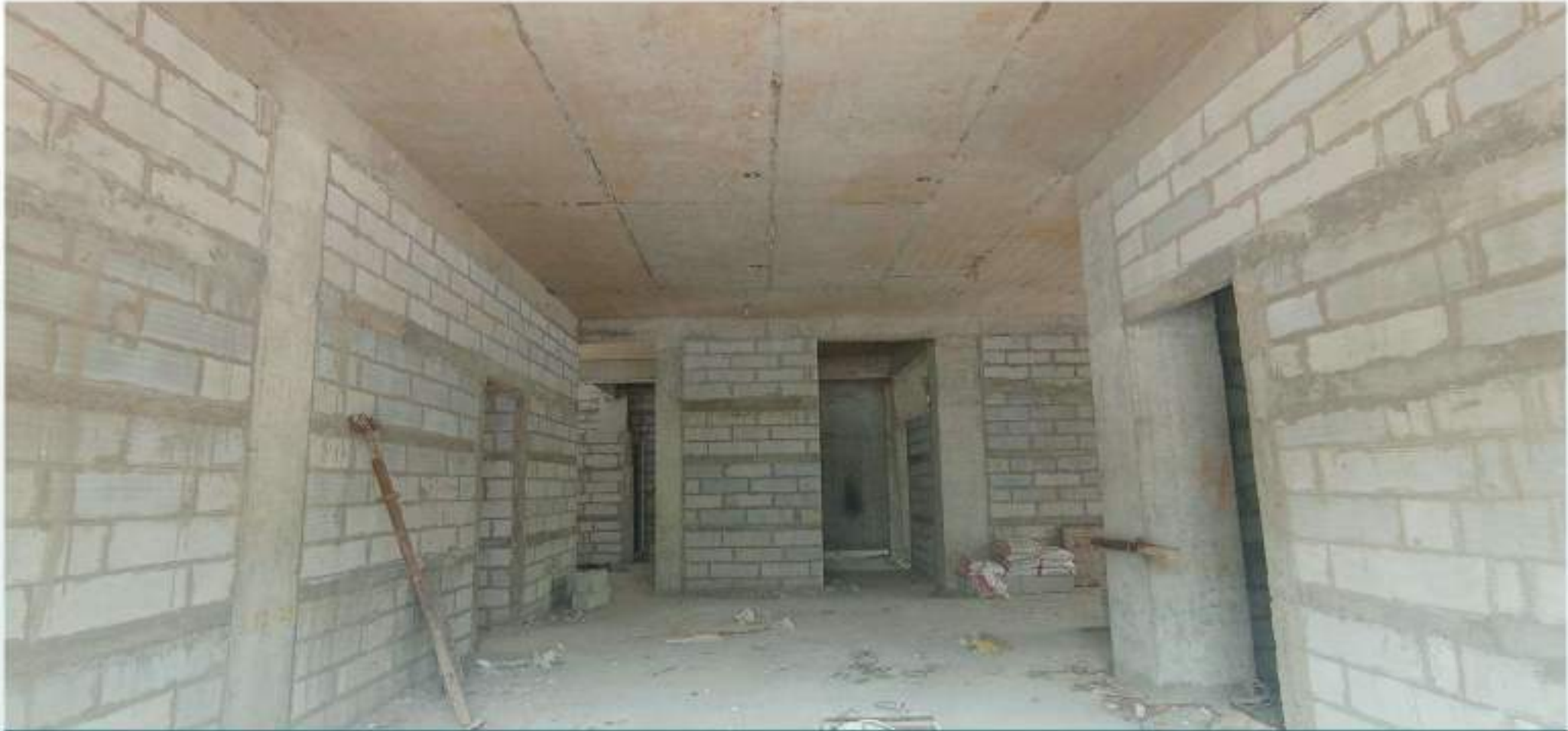
BLOCKWORK AT GROUND FLOOR IN GROUND FLOOR TOWER A
