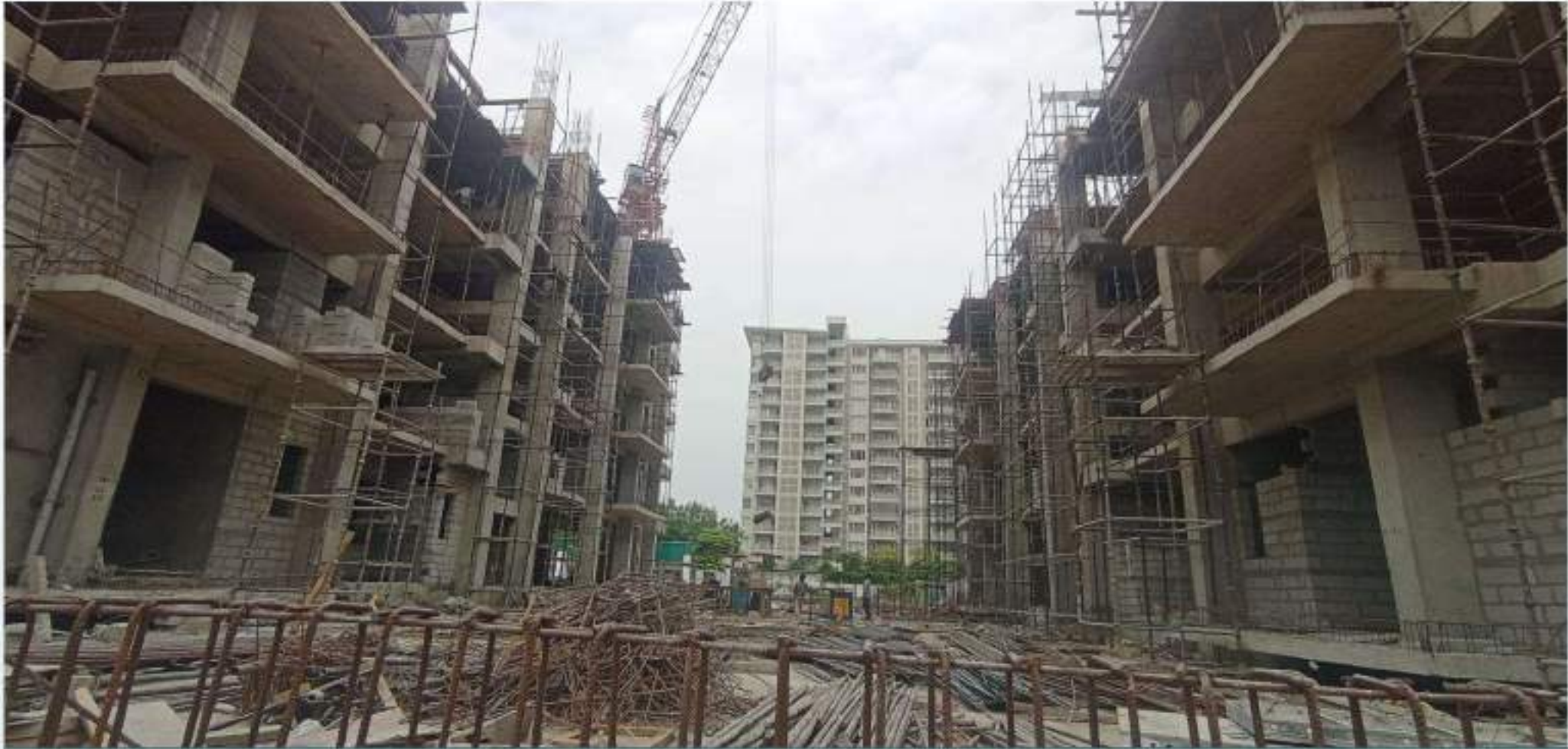
NON TOWER AREA B/W TOWER A & B VIEW FROM RAMP 2
